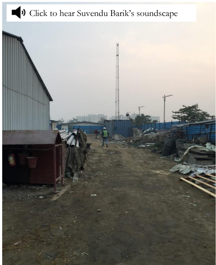
Figure 3. Suvendu Barik’s image of the construction site on campus
